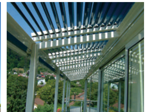
Automatic sun shading system
