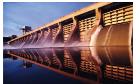
Hydro Power Station / Dam Gates
