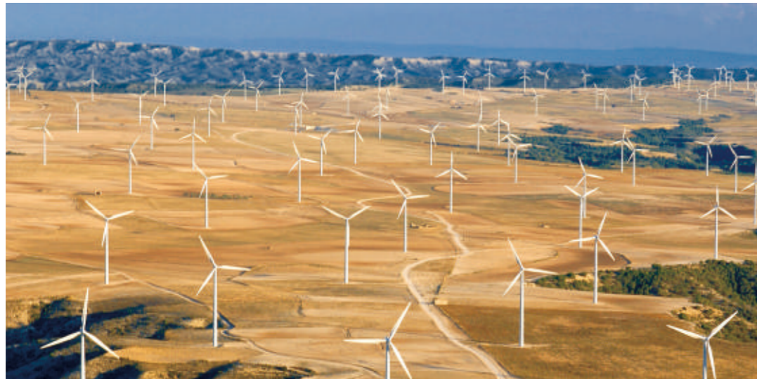
Wind Power Generation
