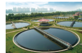
Water treatment facility
